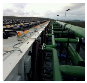
Collectors and electronic motors of the Air Heat Exchangers in detail while working. Each fan motor is provided with a safety switch to allow it's manual shut down.
